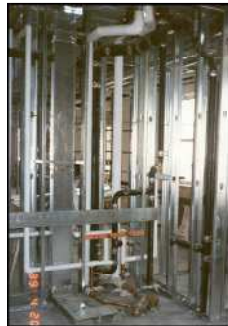
AFTER RE-ROUTING PIPING INTO NEW WALLS
