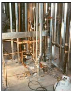
BEFORE RE-ROUTING PIPING INTO NEW WALLS
