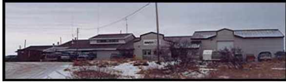
KING SALMON TERMINAL
