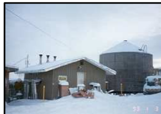
NOATAK WATER TREATMENT PLANT AND VILLAGE WATER STORAGE TANK
